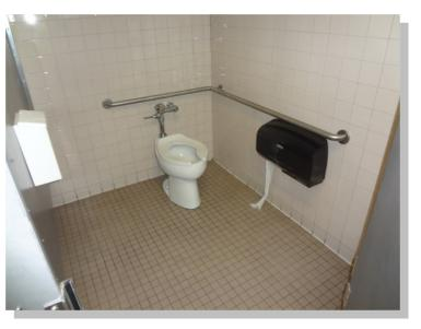
Photo -2 Many of the bathrooms have been upgraded to meet current accessibility standards.
